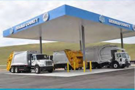
CNG Station - Seminole Road Landfill
