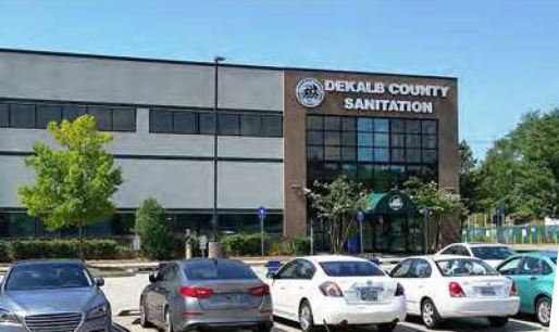
Sanitation Division Administrative Office
