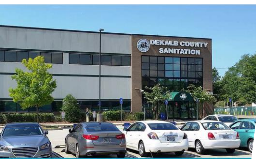
Sanitation Division Administrative Office
