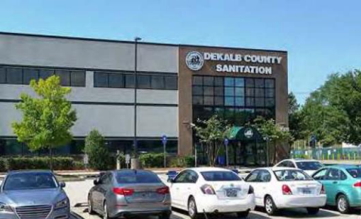
Sanitation Division Administrative Office
