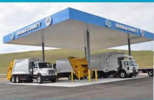
CNG Station - Seminole Road Landfill
