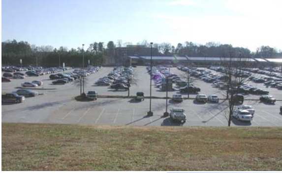
Existing Parking Lot
