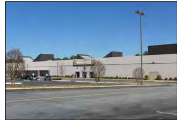
Total Grace Christian Center converted from a big box retail in a shopping area along the corridor
