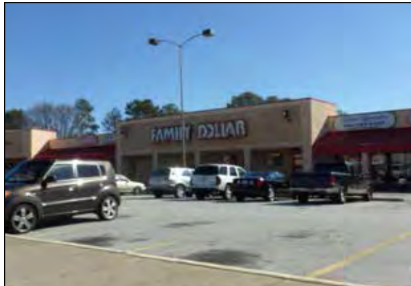
Auto-oriented commercial uses on large parcels are common in the study area corridor
