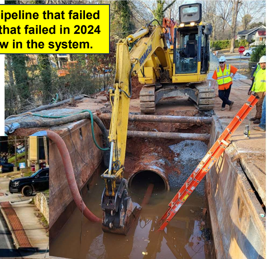
McLendon Road 42" diameter Feb/April 2024 Prestressed Concrete
