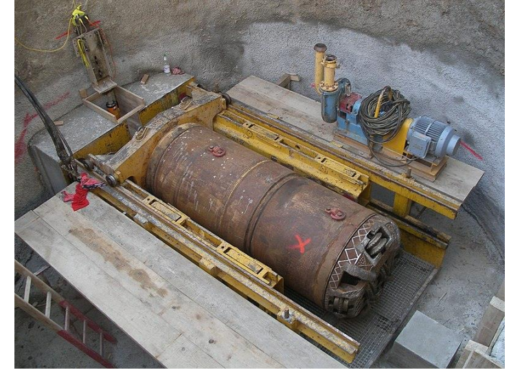
Jack and Bore and Micro Tunneling Under Major Highway/Interstate/GDOT Crossing
