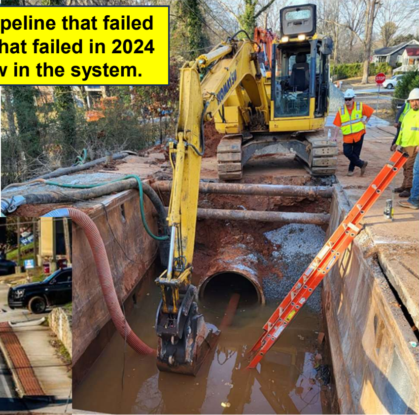
McLendon Road 42" diameter Feb/April 2024 Prestressed Concrete
