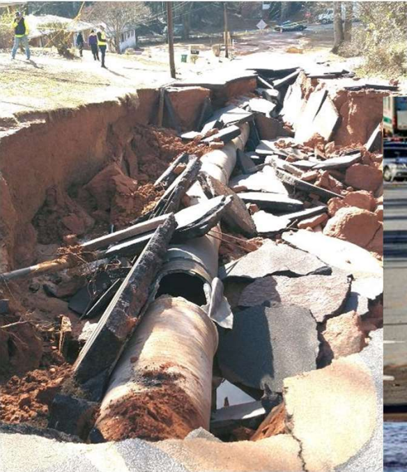
Celia Way January 2023 Prestressed Concrete
