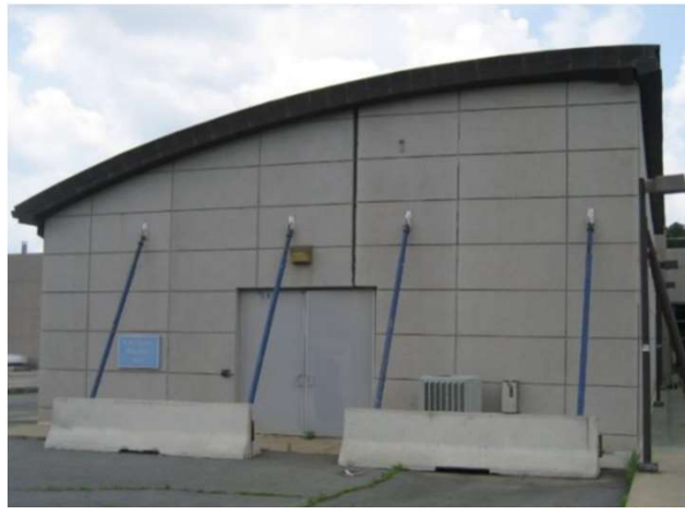
Electrical Building at Water Treatment Plant
