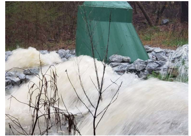
Sanitary Sewer Overflow
