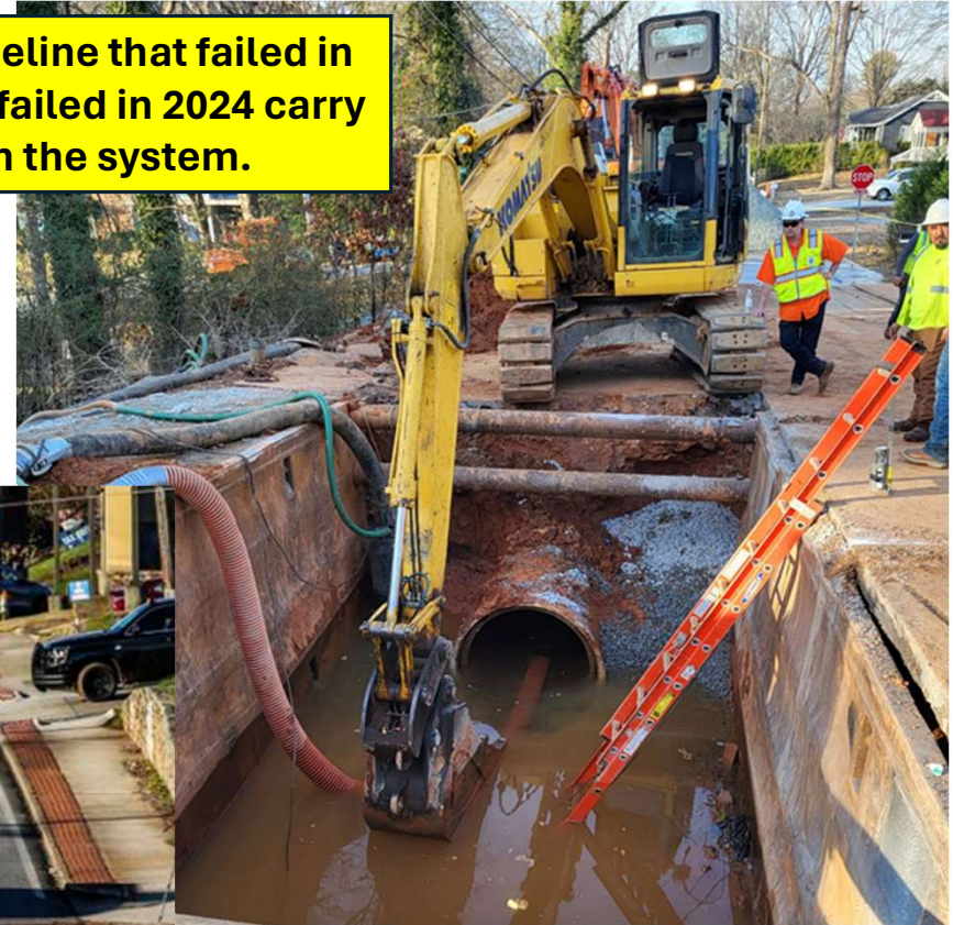
McLendon Road 42" diameter Feb/April 2024 Prestressed Concrete
