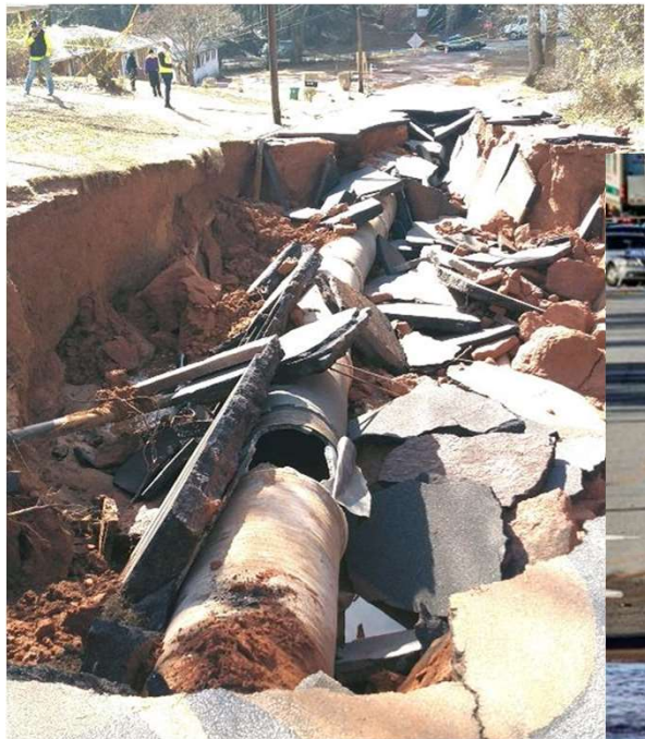
Celia Way January 2023 Prestressed Concrete
