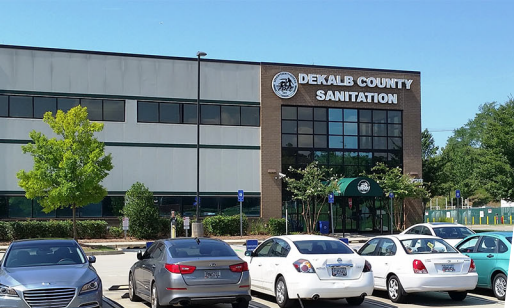
Sanitation Division Administrative Office
