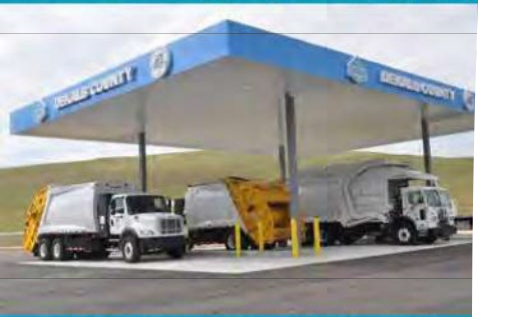
CNG Station – Seminole Road Landfill
