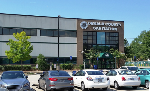
Sanitation Division Administrative Office
