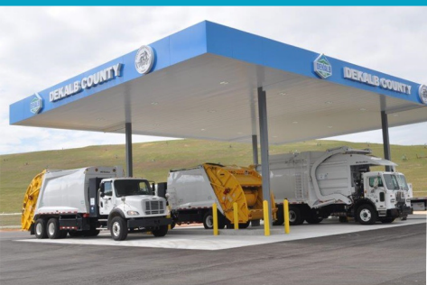
CNG Station – Seminole Road Landfill
