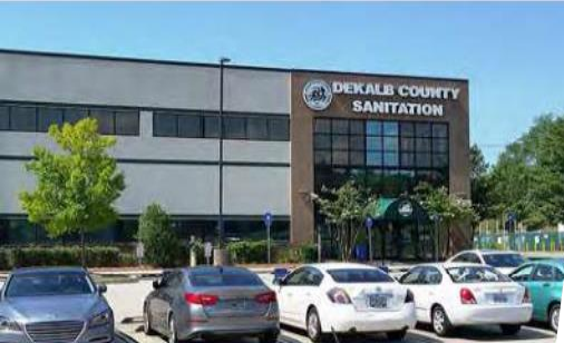
Sanitation Division Administrative Office
