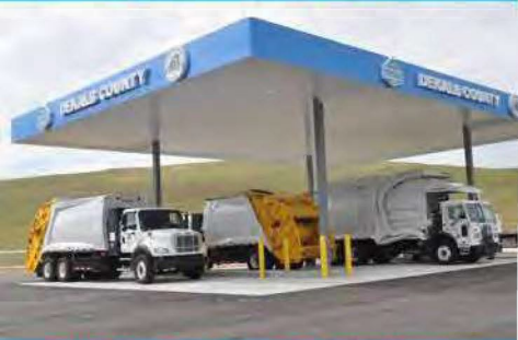
CNG Station – Seminole Road Landfill
