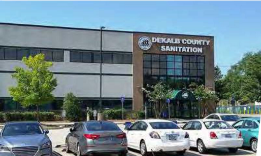
Sanitation Division Administrative Office
