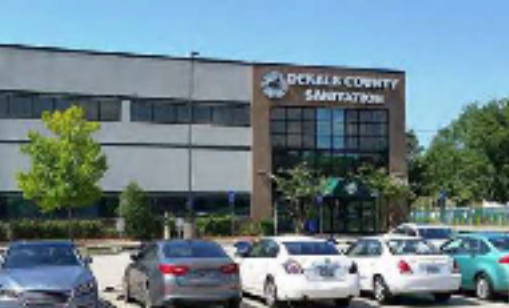
Sanitation Division Administrative Office
