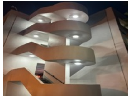
Courthouse Parking Deck
