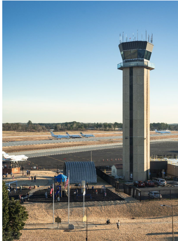
Figure 4-11: PDK Air Traffic Control Tower
