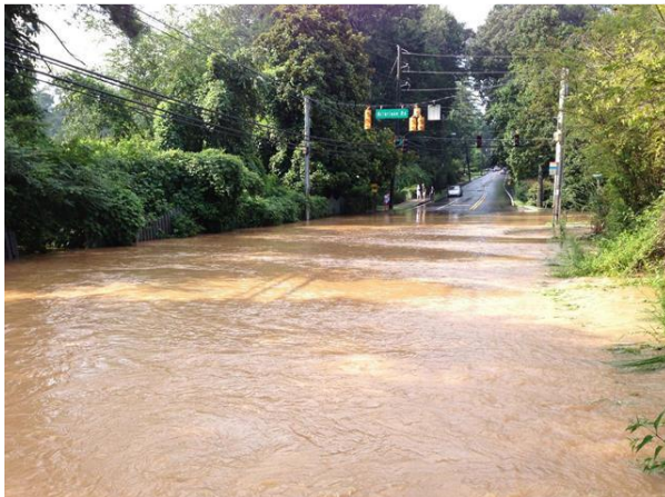
FIGURE 1. Briarcliff Road frequently overtops during minor and major storm events, as shown in this image taken on August 10, 2013.
