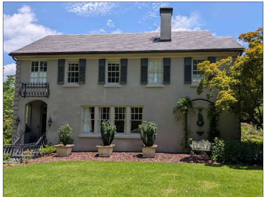
FRONT ELEVATION HISTORIC HOME - NO WORK
