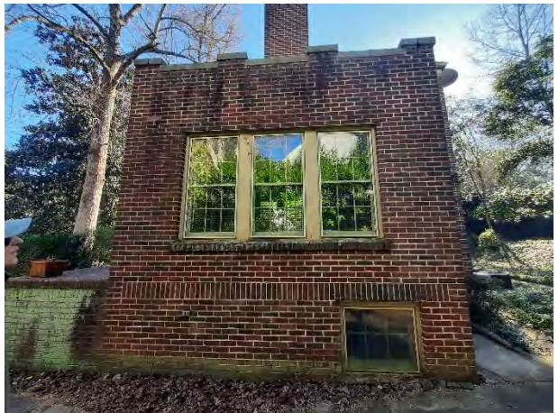
Photo 4 Sunroom / Enclosed Porch (North Façade)
