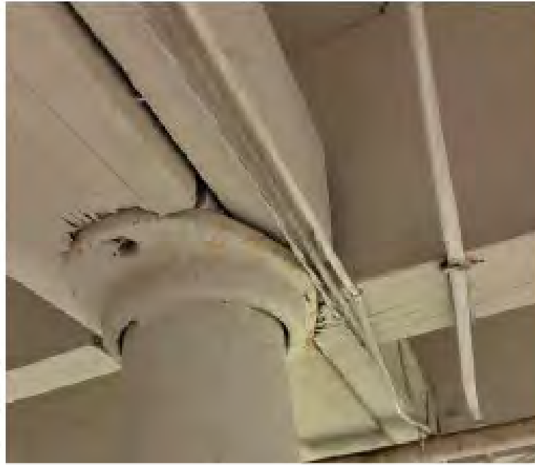
Pillar Foundation Columns No Longer Bearing the Load
