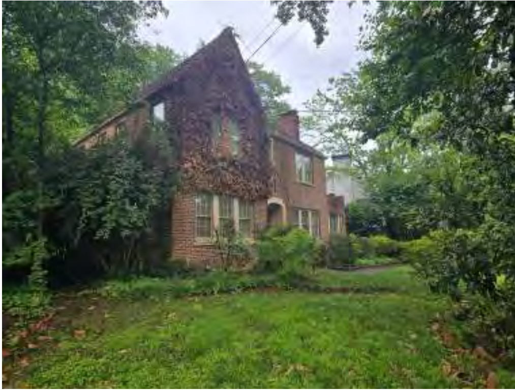
Photo 5 Southeast Corner Elevation with Dense Vegetation ant South Wall
