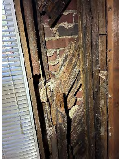
Photo 44 Northwest Corner Framing At Sunroom / Enclosed Porch
