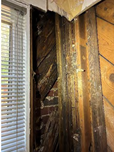
Photo 43 Northwest Corner Framing At Sunroom / Enclosed Porch
