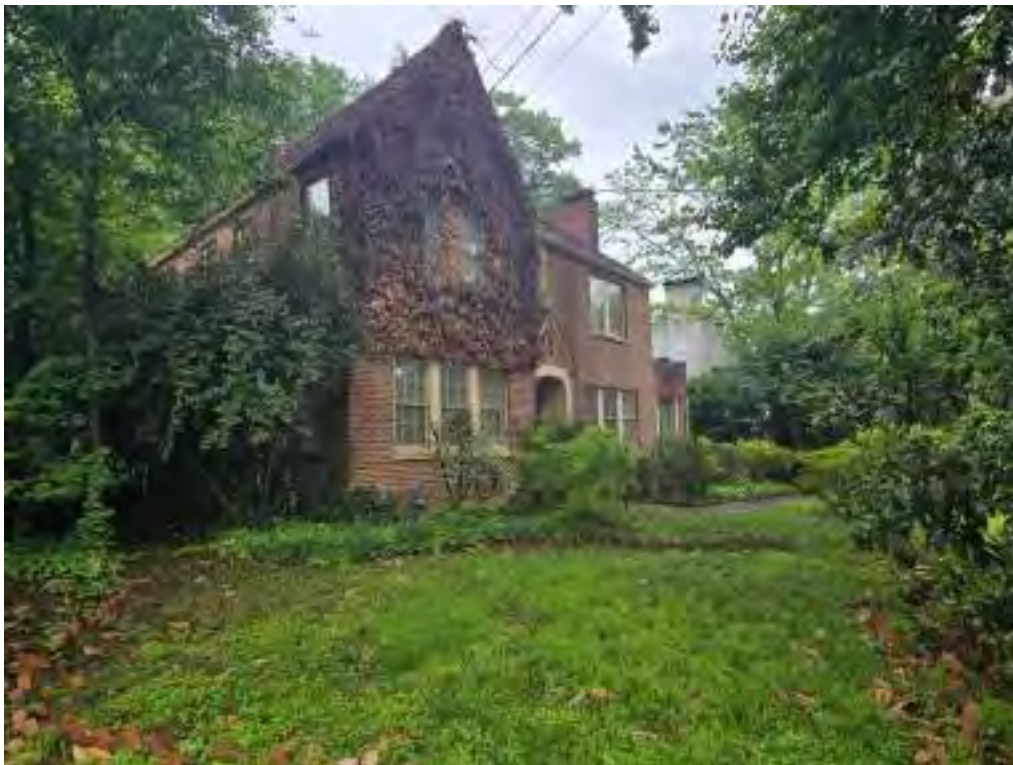
Photo 4 Southeast Corner Elevation with Ivy Coverage at East Front Wall
