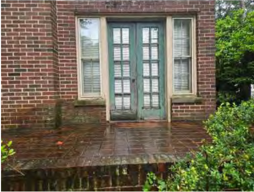
Photo 9 East Elevation with Sunroom Entry and Front Porch
