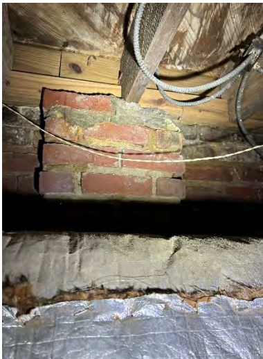
Photo 34 Brick Pilaster at Crawlspace
