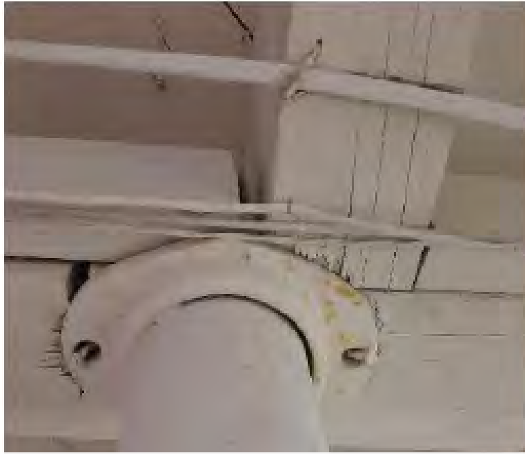
Pillar Foundation Columns No Longer Bearing the Load
