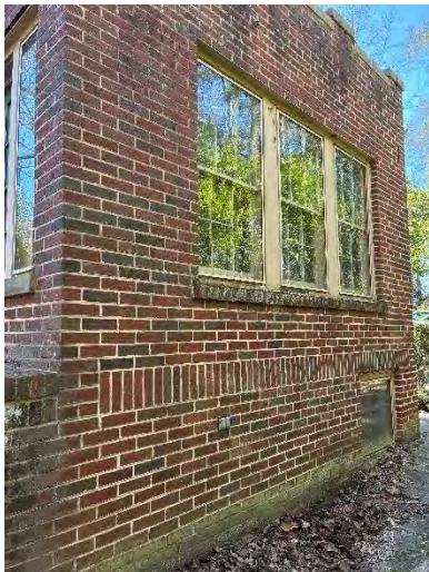
North Exterior Wall of Sunroom / Enclosed Porch
