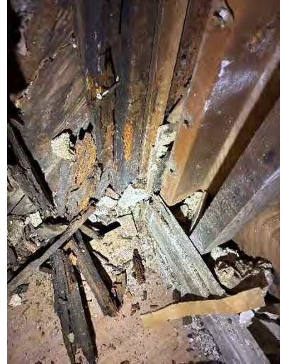
Photo 45 Northwest Corner Framing At Sunroom / Enclosed Porch
