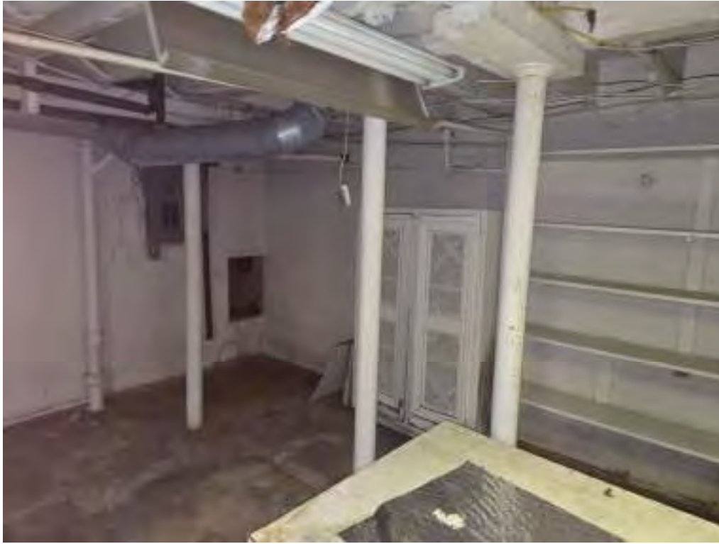
Photo 27 Floor Framing and Interior Posts Southeast Corner of Basement
