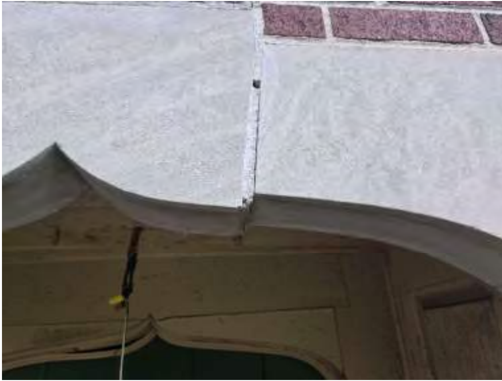
Photo 13 Front Entry Door Vestibule With Dropped Stone Pediment
