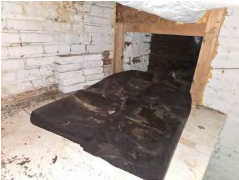
Photo 32 Access Passage to Crawl Space Below Front Entry Porch
