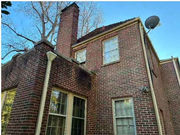
Photo 3 North Side of House
