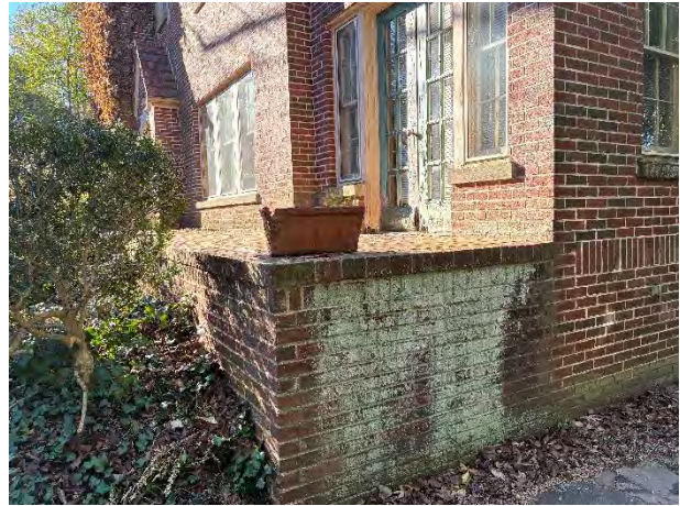
Northeast Corner of Exterior Patio
