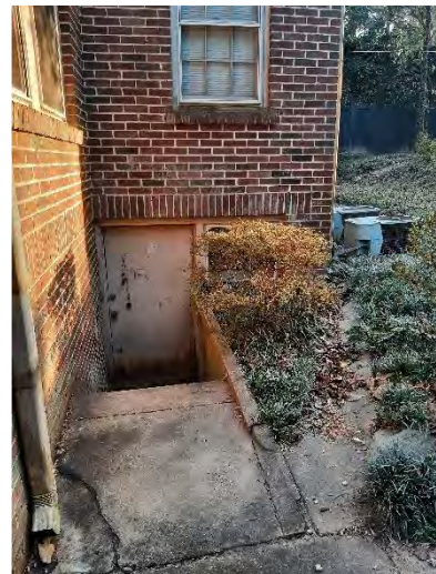
Photo 38 Exterior Basement Entrance
