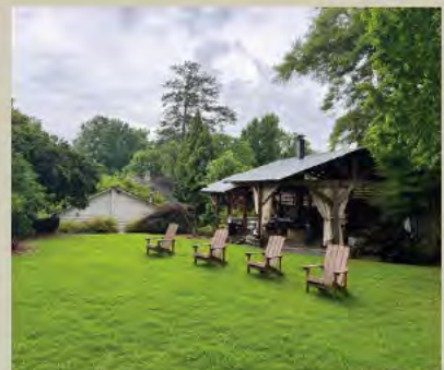
Rear View of Deck
