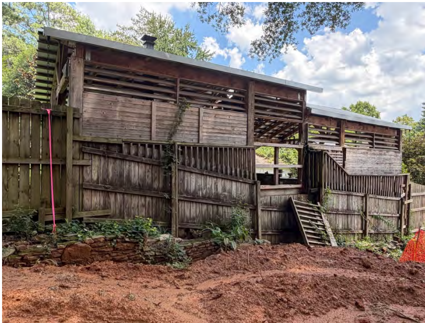
View of 1194's 880-square-foot structure from 1190 Clifton.
