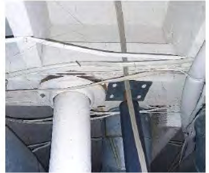
Pillar Foundation Columns No Longer Bearing the Load
