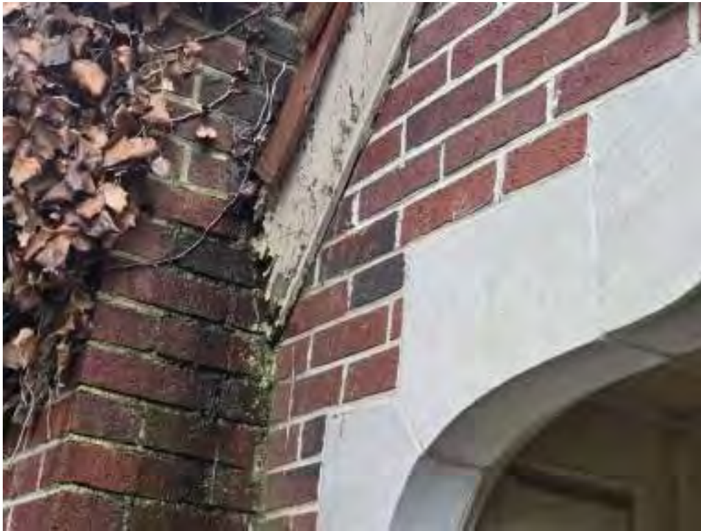
Photo 11 East Elevation with Front Entry Door Vestibule Pediment and Cornice
