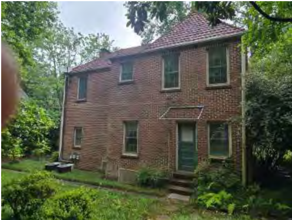
Photo 6 West Elevation with Kitchen Entrance
