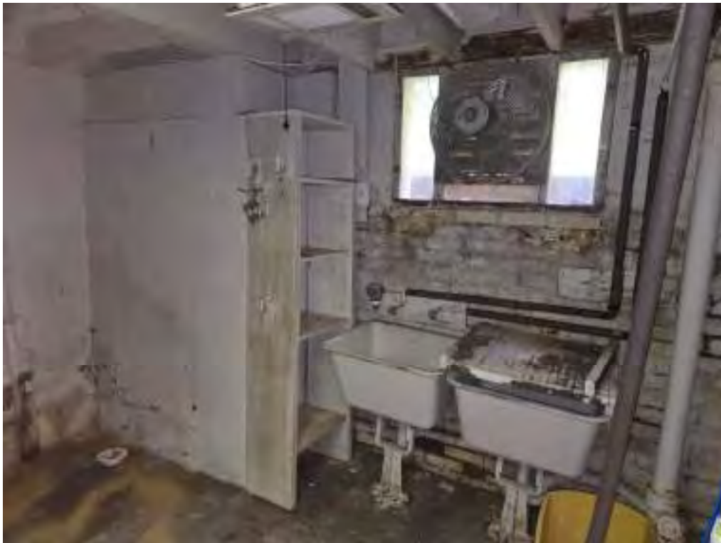
Photo 28 Floor Framing and Interior Posts Southwest Corner of Basement
