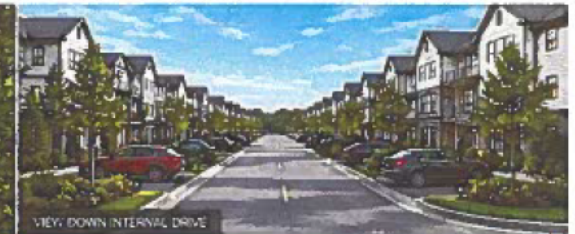
VIEW DOWN INTERNAL DRIVE
