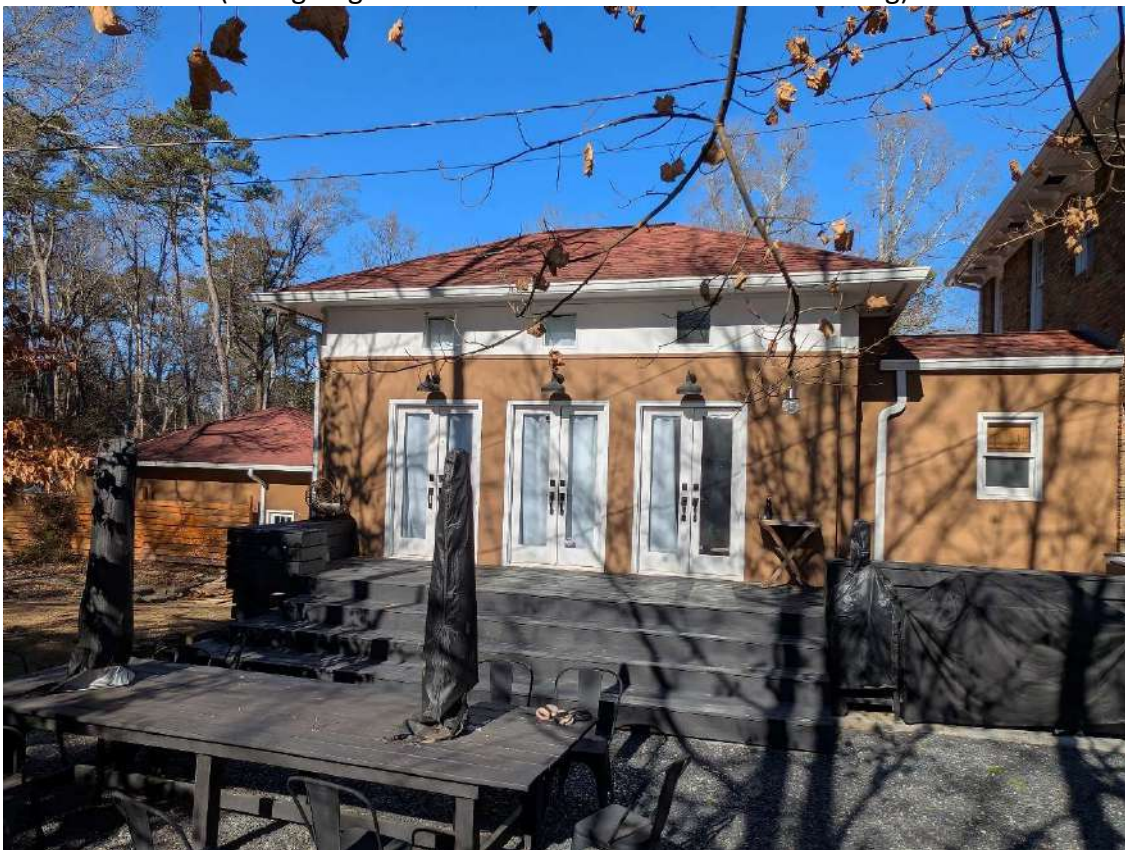
Existing non-historic stucco rear addition from the left side
