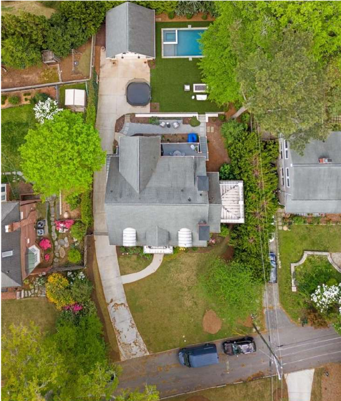
Aerial view of home.
