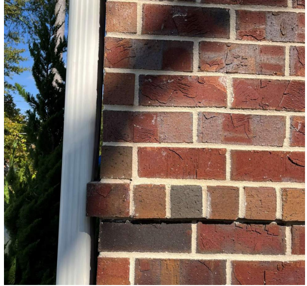
New modular, red brick to match existing.
