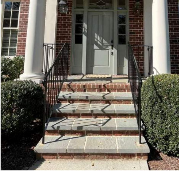
New bluestone pavers to match existing.
