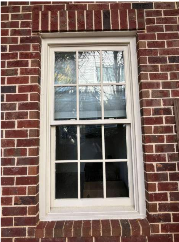
New brick headers to match existing.
