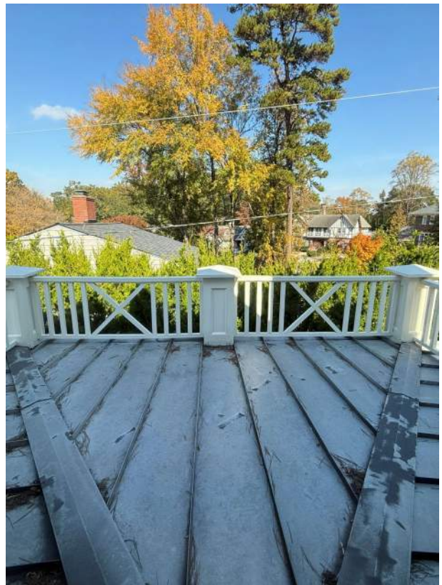
New metal standing seam roof to match existing.
