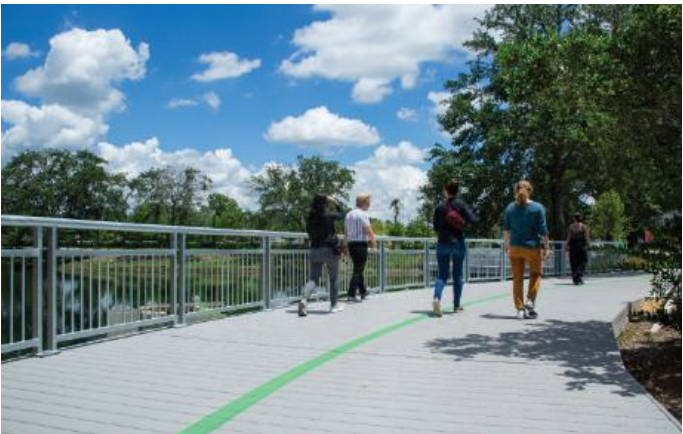
FIGURE 53 - LEFT: EMERALD TRAIL SEGMENT, PHOTOS FOR POND AND COMPANY RIGHT: ATLANTA AREA TRAILS AND GREENWAYS, PHOTOS FOR POND AND COMPANY
