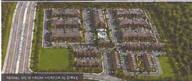
AERIAL VIEW FROM MEMORIAL DRIVE
