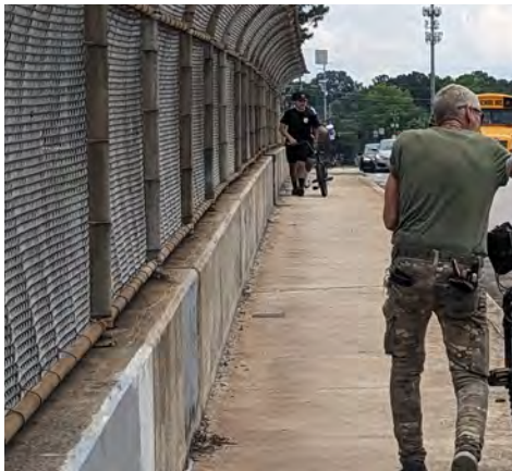
FIGURE 23 - MULTIPLE CYCLISTS CROSSING THE I-285 OVERPASS
