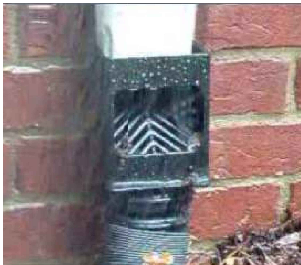
IN-LINE LEAF STRAINER N.T.S.
