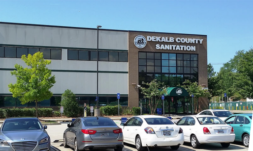
Sanitation Division Administrative Office
