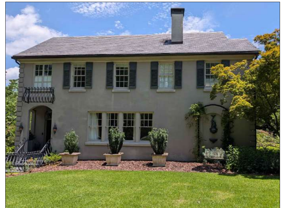
FRONT ELEVATION HISTORIC HOME - NO WORK
