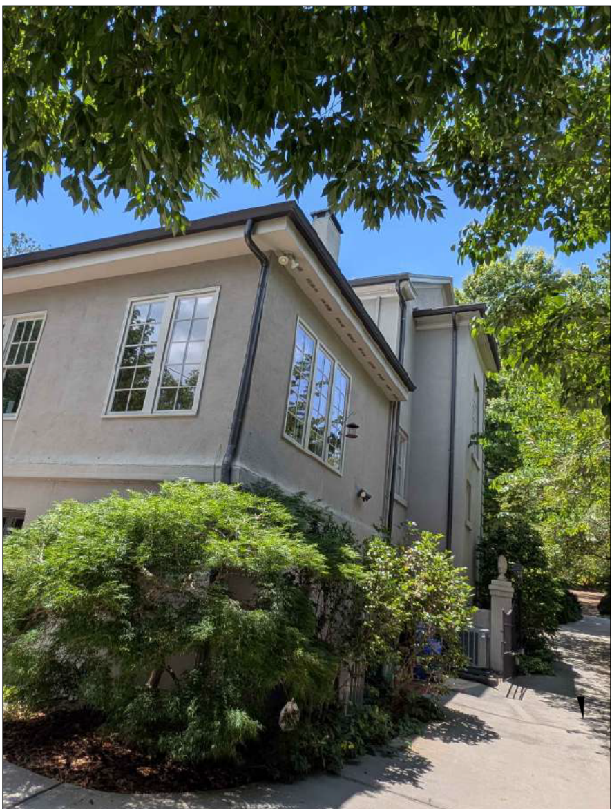
LEFT SIDE ELEVATION AT REAR CORNER
