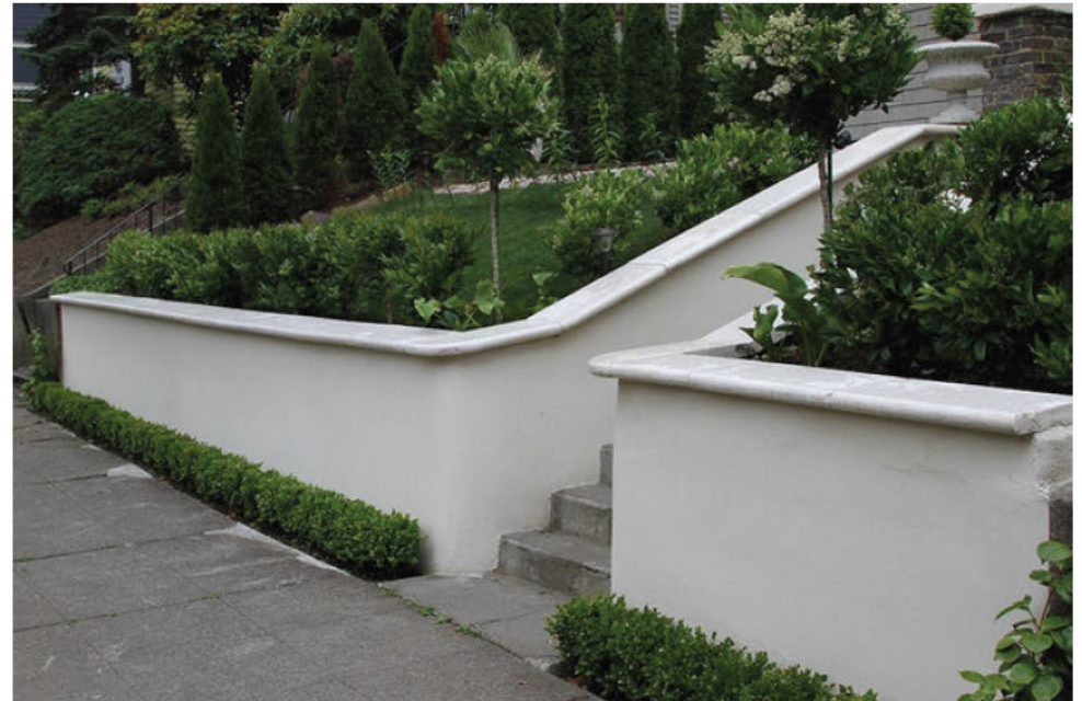
Stucco Retaining Wall
