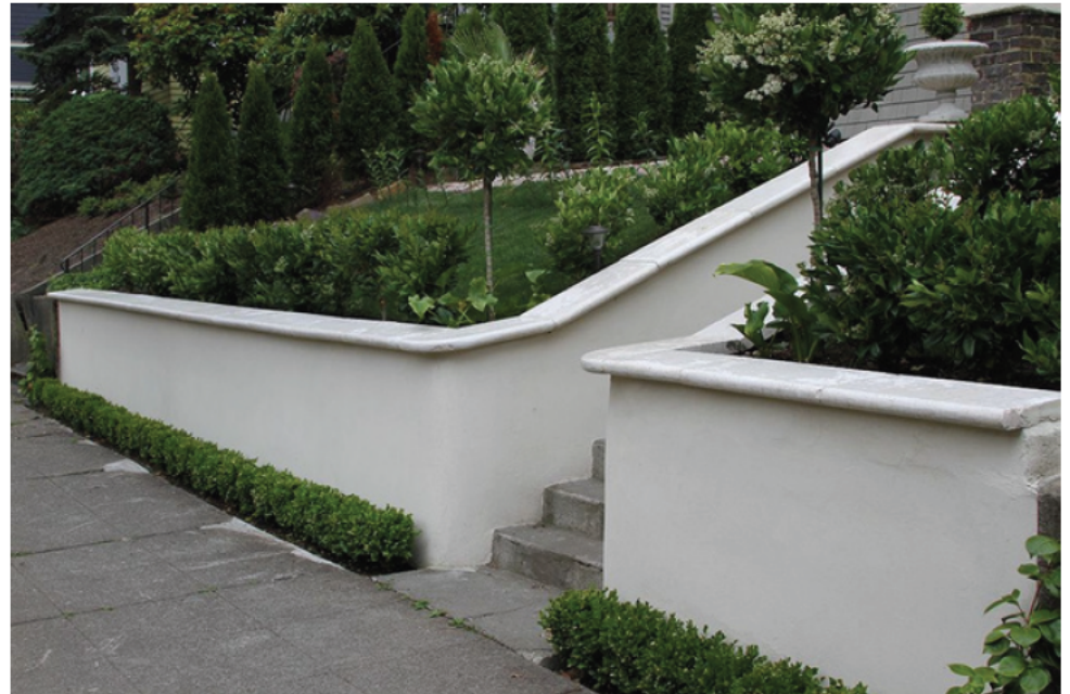
Stucco Retaining Wall
