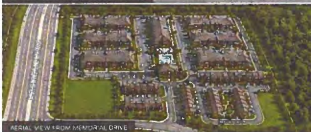
AERIAL VIEW FROM MEMORIAL DRIVE
