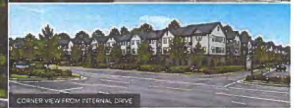
CORNER VIEW FROM INTERNAL DRIVE
