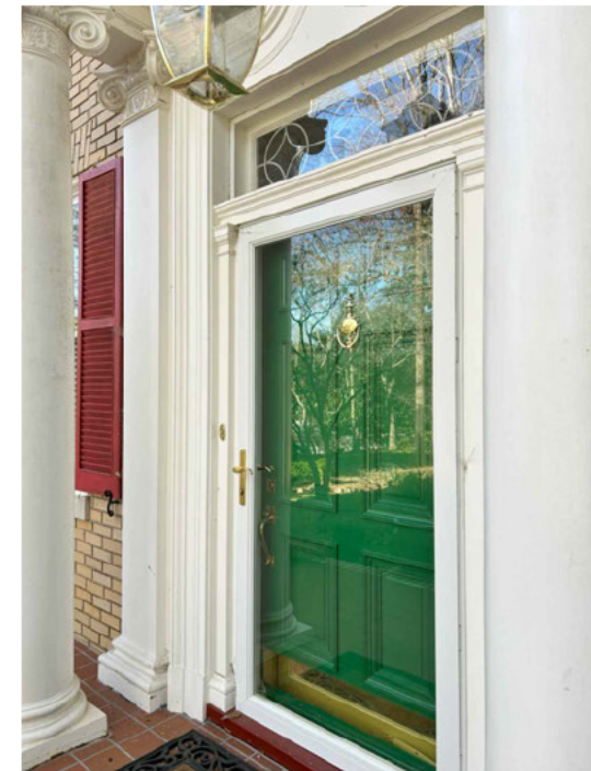
IMAGE 4 EXISTING N. DECATUR RD. ENTRY DOOR. MATCH LEADED GLASS TRANSOM WINDOW DESIGN.
