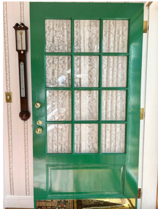
IMAGE 3 EXISTING DRIVEWAY ENTRY DOOR. MATCH RAISED PANEL STYLE AND PAINT COLOR.
