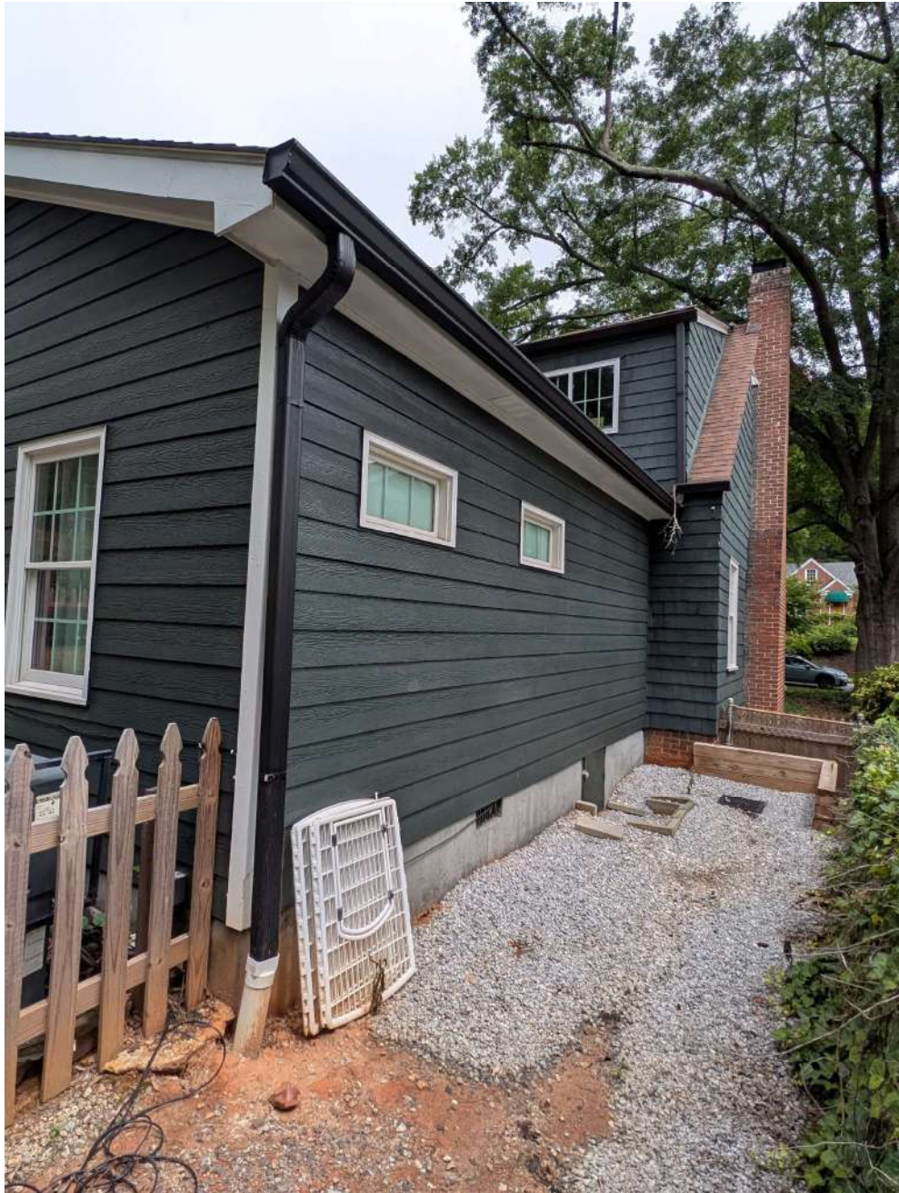
Left side of existing non-historic rear addition where a pair of windows will be added
