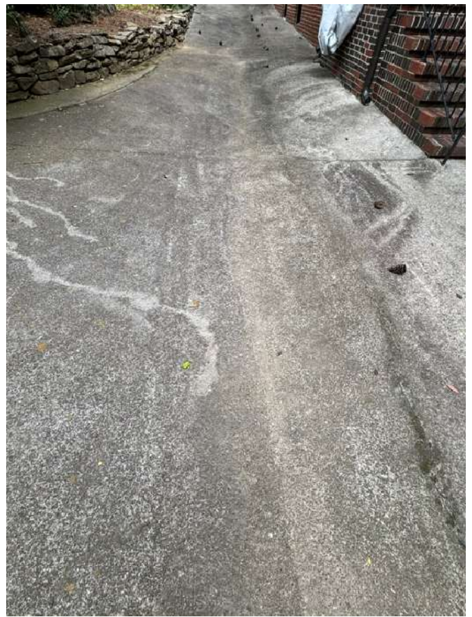
Stains show existing years-old swale in current driveway, making grass strip impractical
