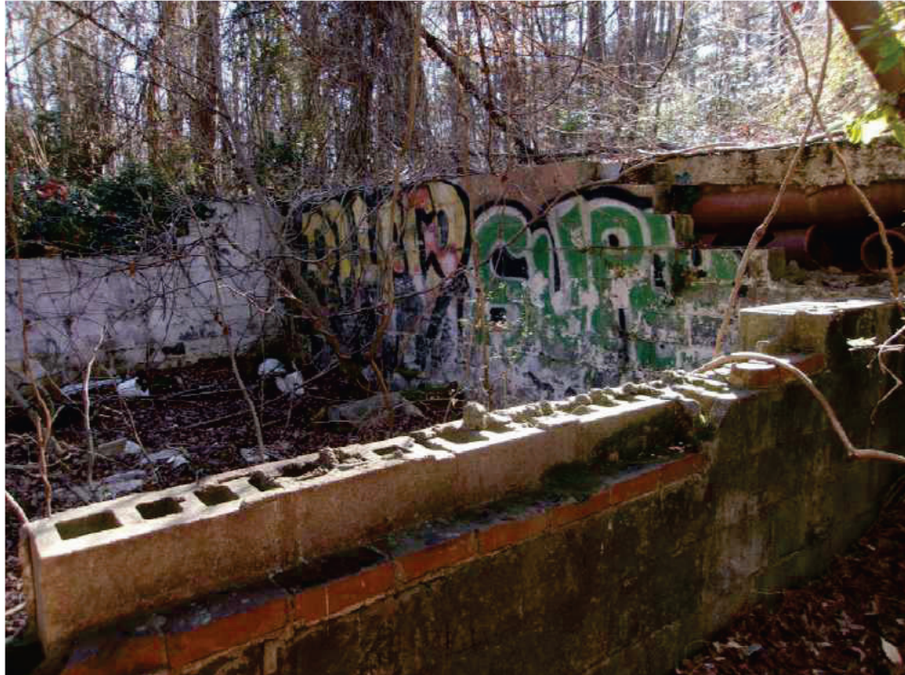
Near Transect 7, Shovel Test, Facing Southwest
