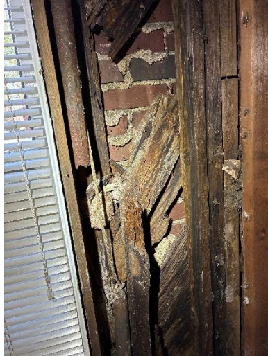
Photo 44 Northwest Corner Framing At Sunroom / Enclosed Porch
