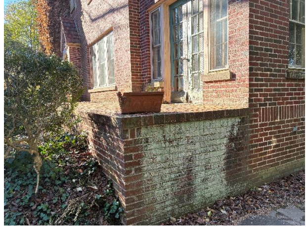
Northeast Corner of Exterior Patio
