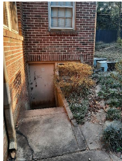
Photo 38 Exterior Basement Entrance
