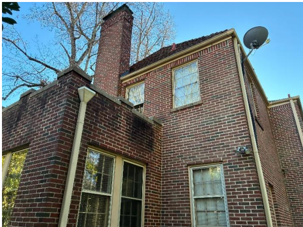
Photo 3 North Side of House
