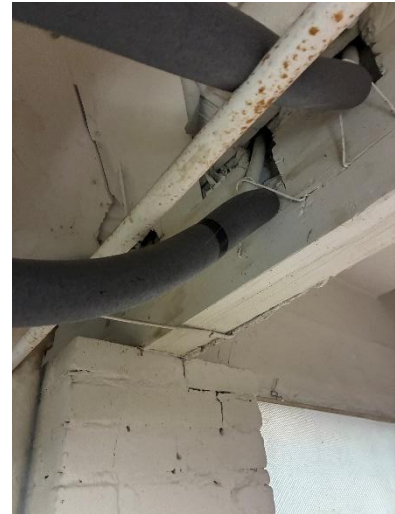
Photo 27 Header Beam at Stair Opening
