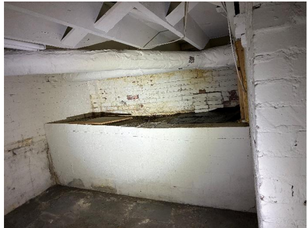
Photo 47 Basement Below Sunroom / Enclosed Porch Showing Floor Framing
