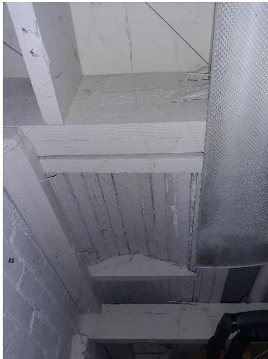
Framing Under Hearth
