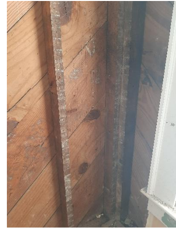
Photo 18 Second Floor Wall
