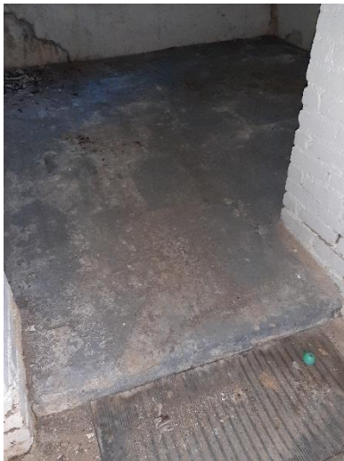
Photo 36 Slab on Grade
