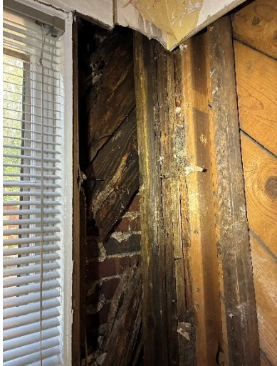
Photo 43 Northwest Corner Framing At Sunroom / Enclosed Porch
