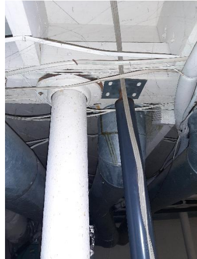
Photo 30 Top of Pipe Column With Adjacent Shoring Post
