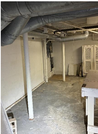
Photo 37 Slab on Grade
