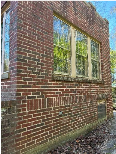
North Exterior Wall of Sunroom / Enclosed Porch
