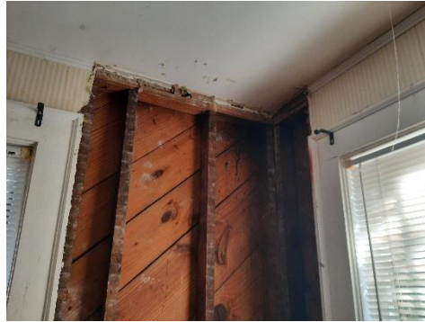
Photo 17 Second Floor Wall
