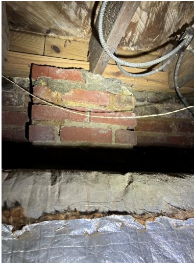
Photo 34 Brick Pilaster at Crawlspace
