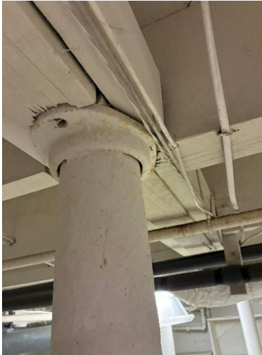
Photo 29 Top of Pipe Column
