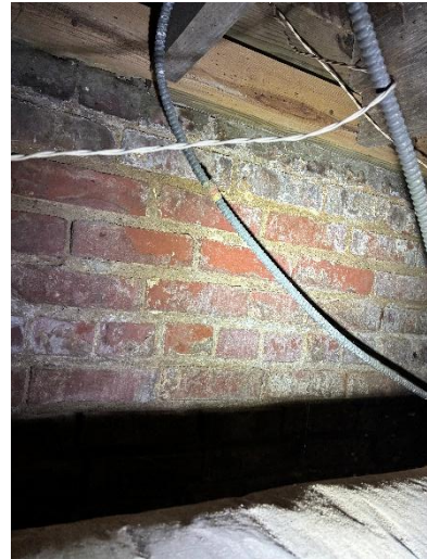
Photo 35 Exterior Wall at Crawlspace
