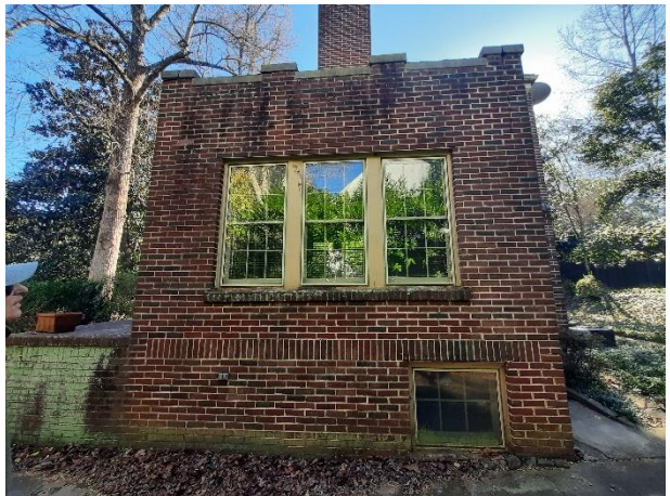
Photo 4 Sunroom / Enclosed Porch (North Façade)
