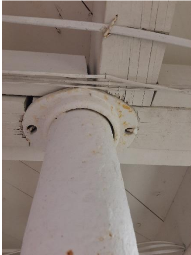
Photo 28 Top of Pipe Column
