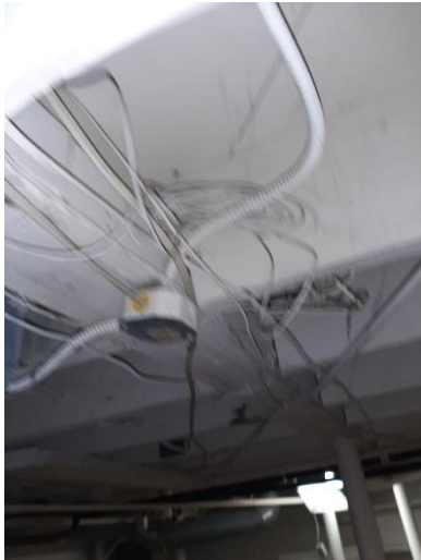
Photo 25 First Floor Framing
