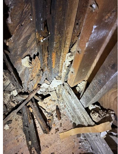
Photo 45 Northwest Corner Framing At Sunroom / Enclosed Porch
