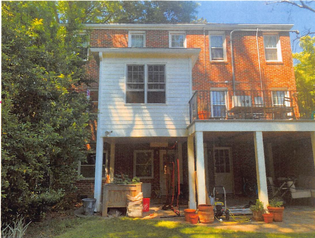
Figure 3: Back kitchen window sash to be replaced
