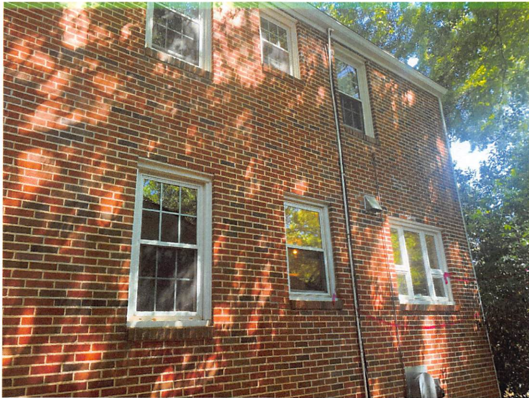
Figure 4: Side kitchen window sashes to be replaced
