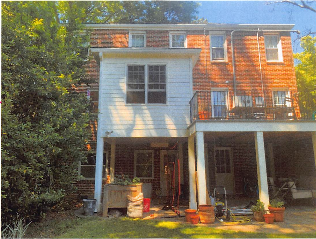
Figure 3: Back kitchen window sash to be replaced
