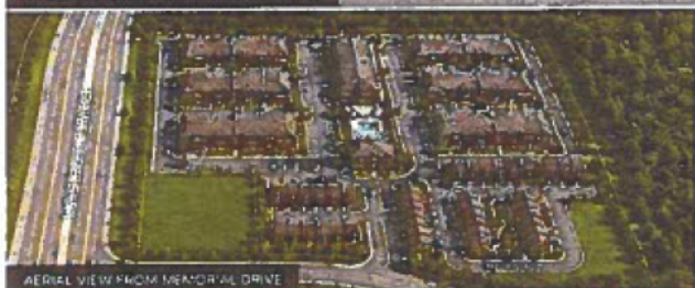
AERIAL VIEW FROM MEMORIAL DRIVE
