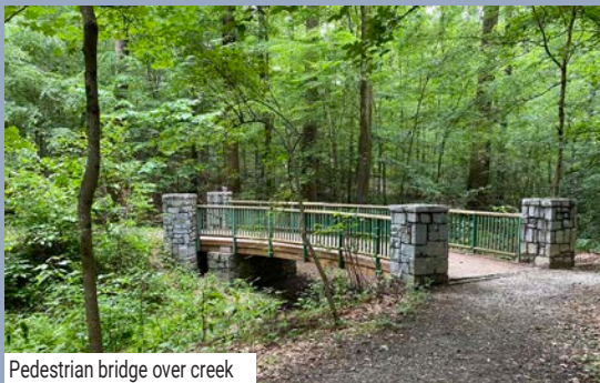
Pedestrian bridge over creek
