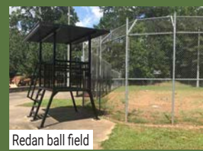
Redan mixed-use field and grandstand
