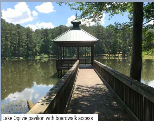
Lake Ogilvie pavilion with boardwalk access
