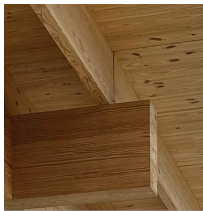
SOUTHERN YELLOW PINE RAFTERS & ROOF SOFFIT CLADDING
