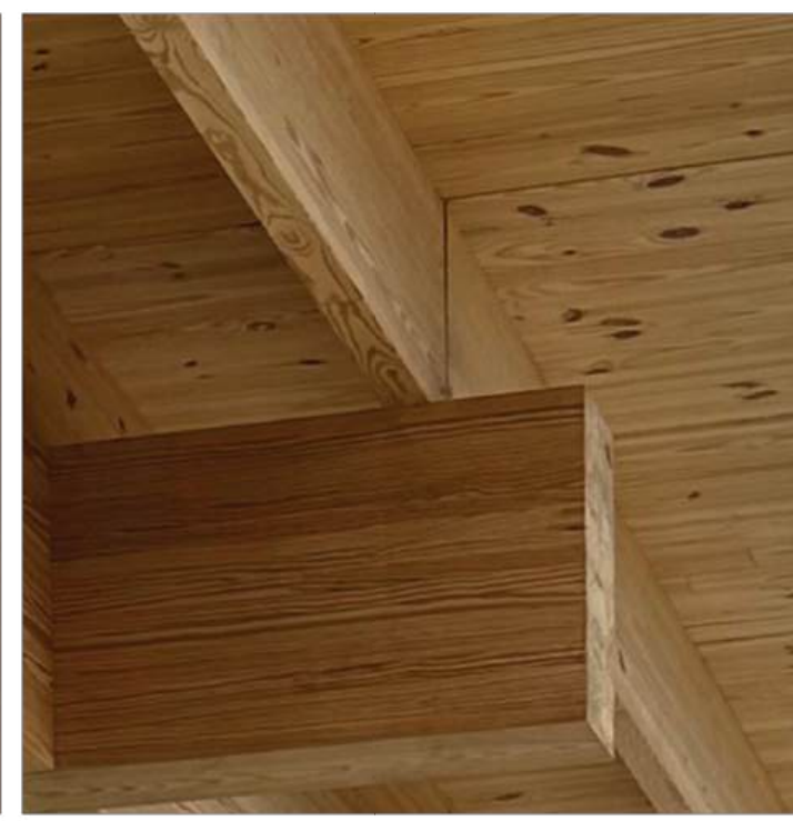
SOUTHERN YELLOW PINE RAFTERS & ROOF SOFFIT CLADDING
