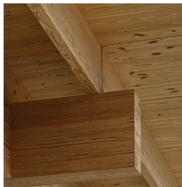
SOUTHERN YELLOW PINE RAFTERS & ROOF SOFFIT CLADDING
