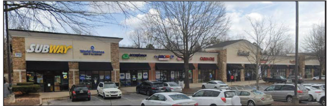
OVERALL VIEW OF FLAT SHOALS CROSSING
