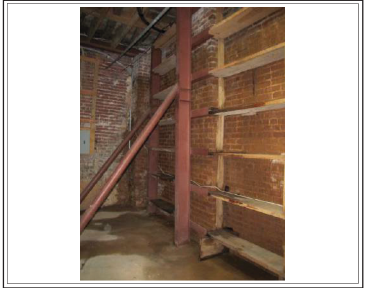
Basement Structure Reinforcement
