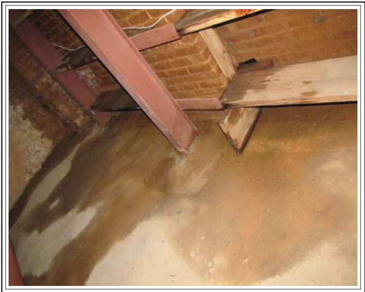
Basement Structure Reinforcement
