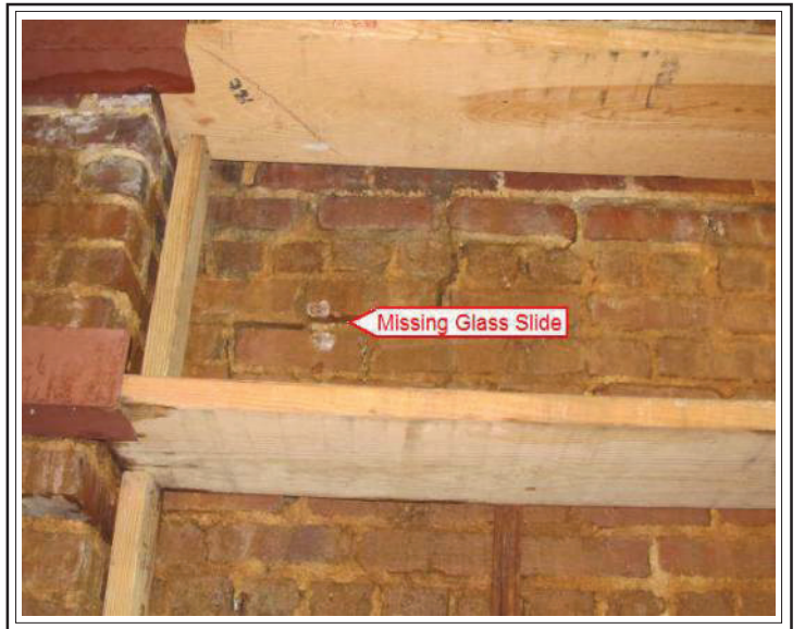
Basement Structure Reinforcement
